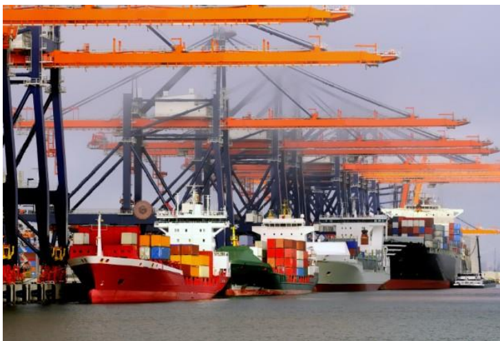
A typical container cargo terminal
