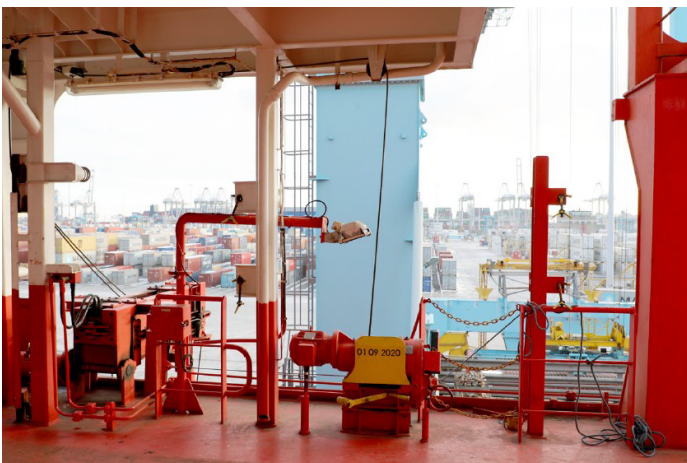
Ref DMAIB Report 10/05/2021 – Site of incident
