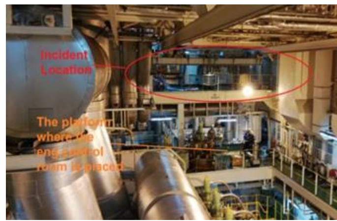
Platform where blowers were stowed (red) – ( Ref TMSI Report: 18/2019 )
