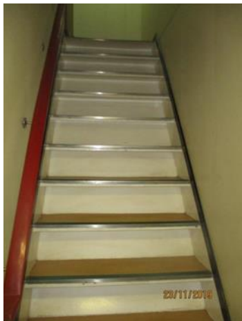
Stairway (Ref: TMSI Report: 22/2020)
