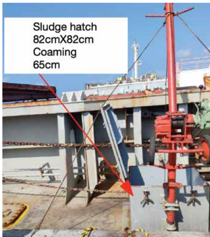
Sludge hatch and mucking winch
