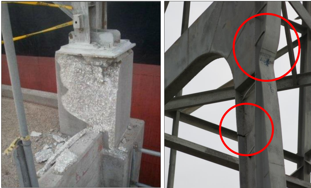
Close-up of a damaged concrete pedestal (left) at the Louis Dreyfus Grain Elevator and a cracked weld and bent I-beam on a vertical support (right). (Left photo by Coast Guard)
