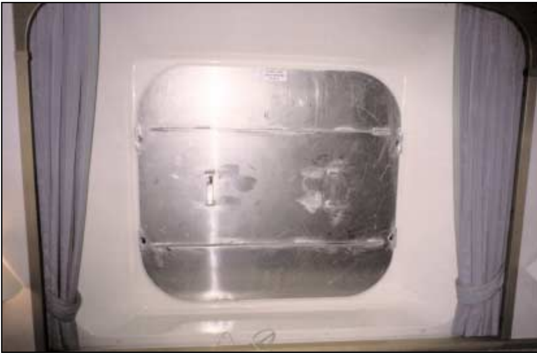
Photograph of storm cover in position
