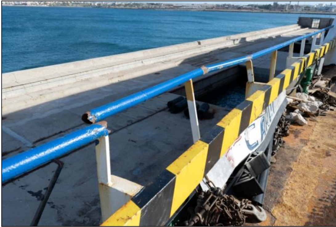
Figure 23: Damaged guard rails
