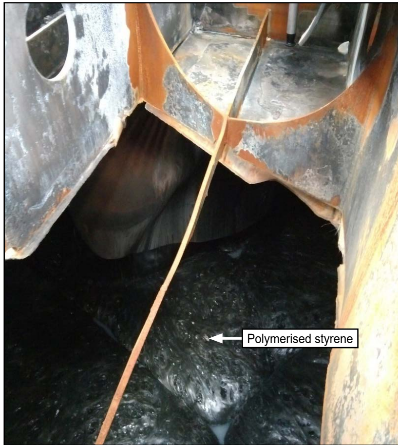
Figure 12: 9S tank rupture
