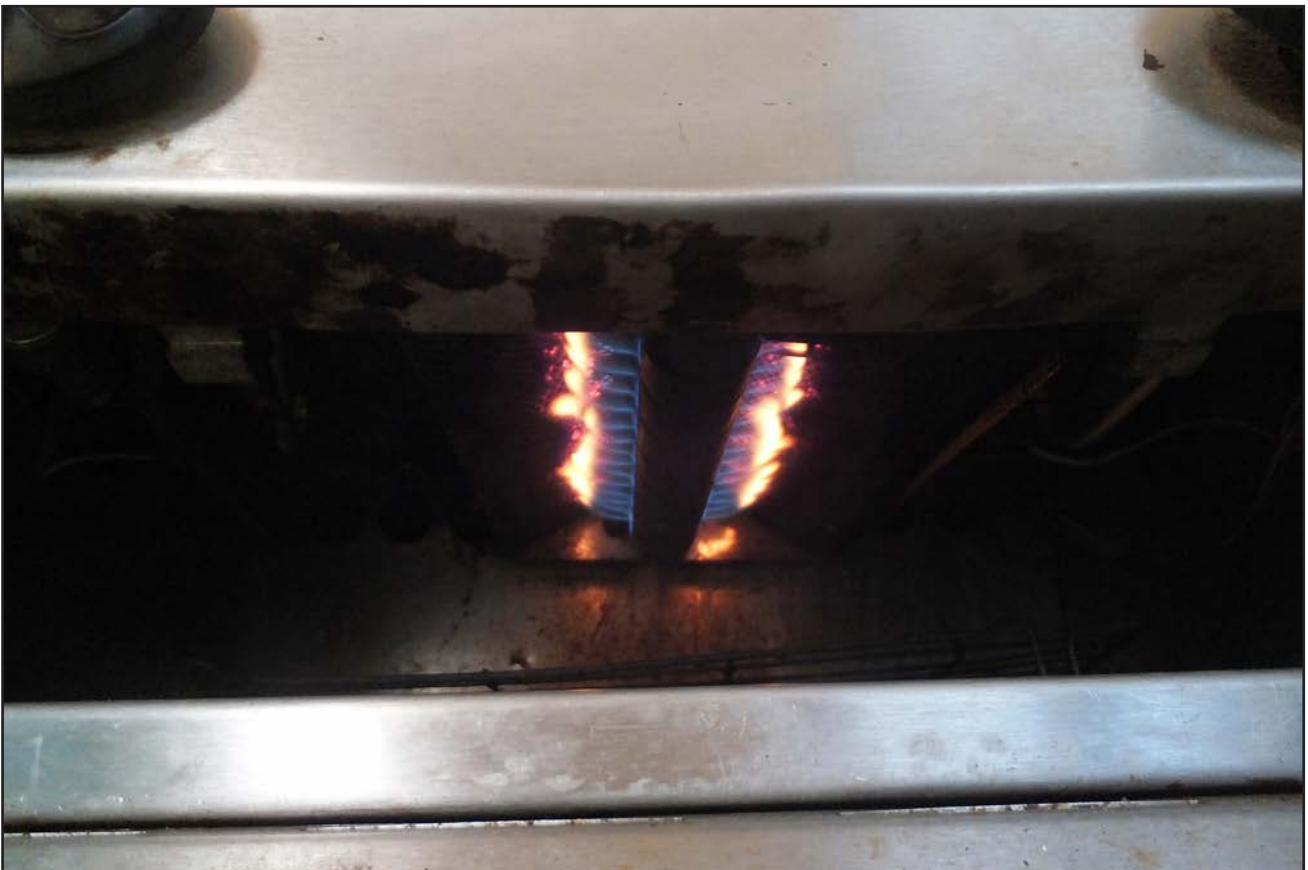
Corroded grill
