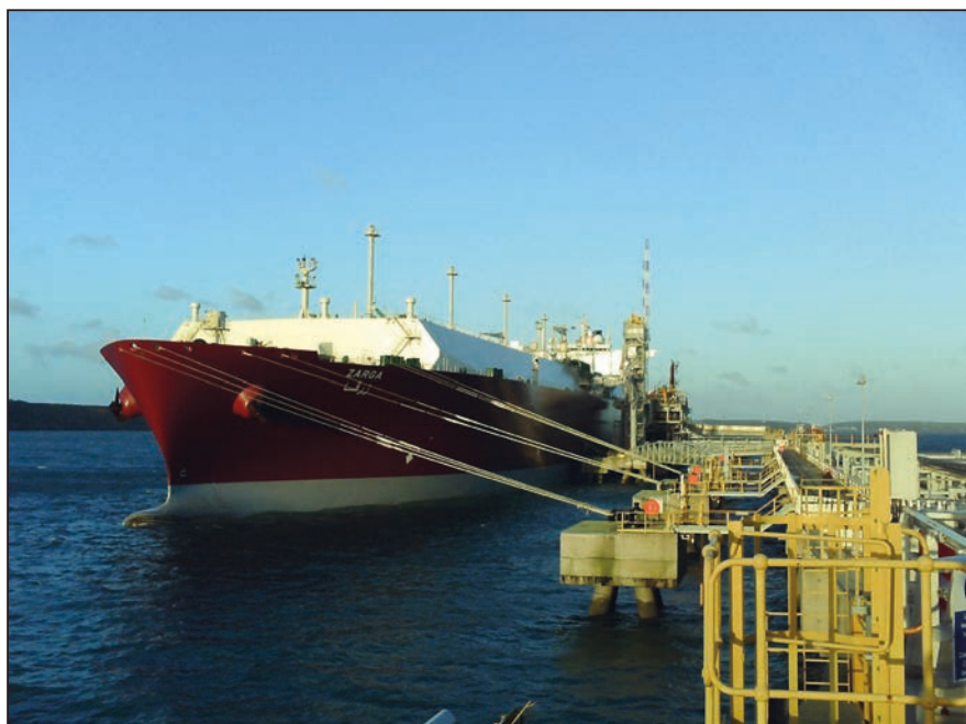
Figure 1: Zarga alongside South Hook LNG terminal
