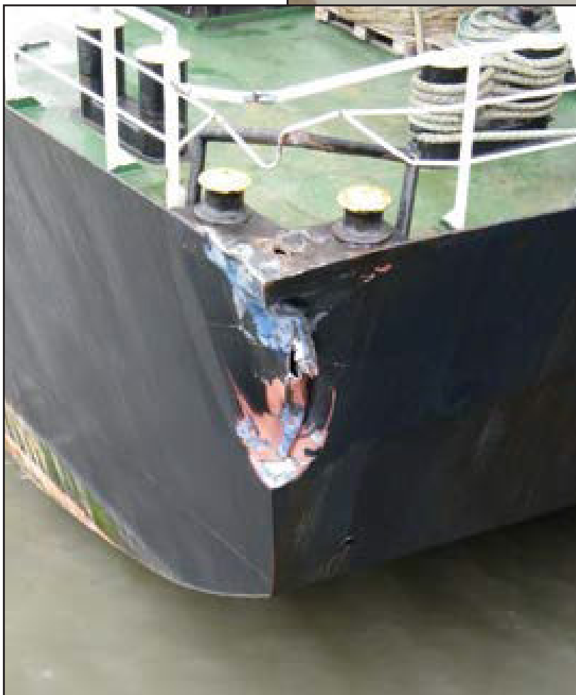
Figure 3: Damage to shell plating
