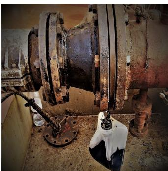
Drip sampler and sealed container
