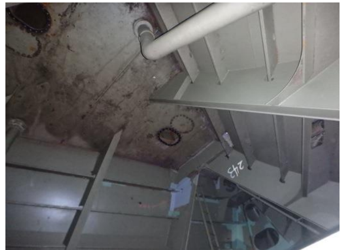
Inaccessible side tank covers
