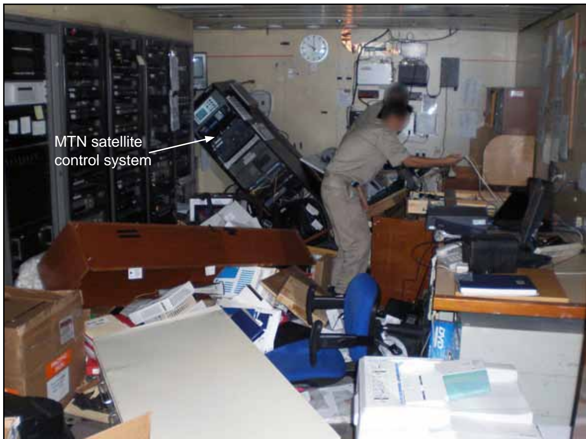
Electro Technical Office after the accident
