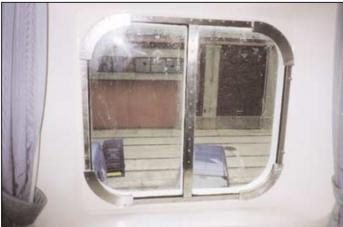
Photograph of window fitted with retaining plates
