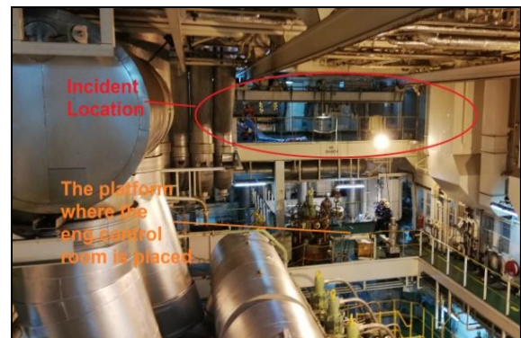
Figure 13: Platform where blowers were stowed (red)
